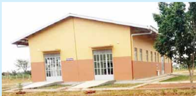
Plumbing workshop at Kasodo Technical Institute. PHOTO/ COURTESY
